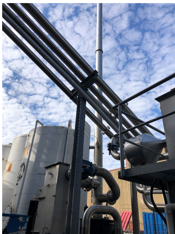
Image 2 – EPA 2 Vapour Scrubber Stack
